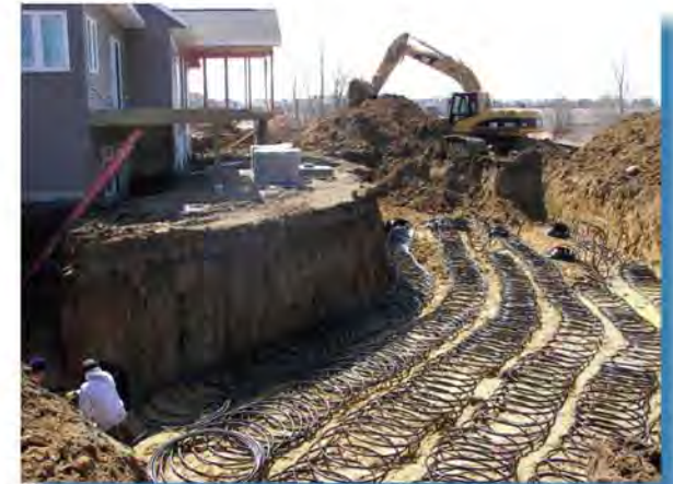
A typical horizontal slinky loop installation
