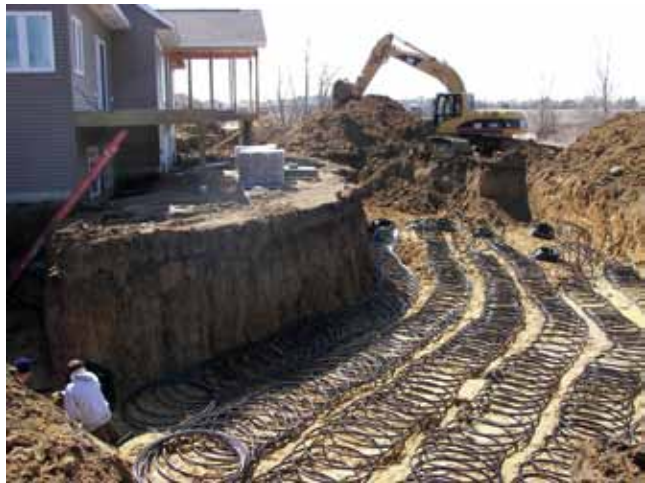
A typical horizontal slinky loop installation
